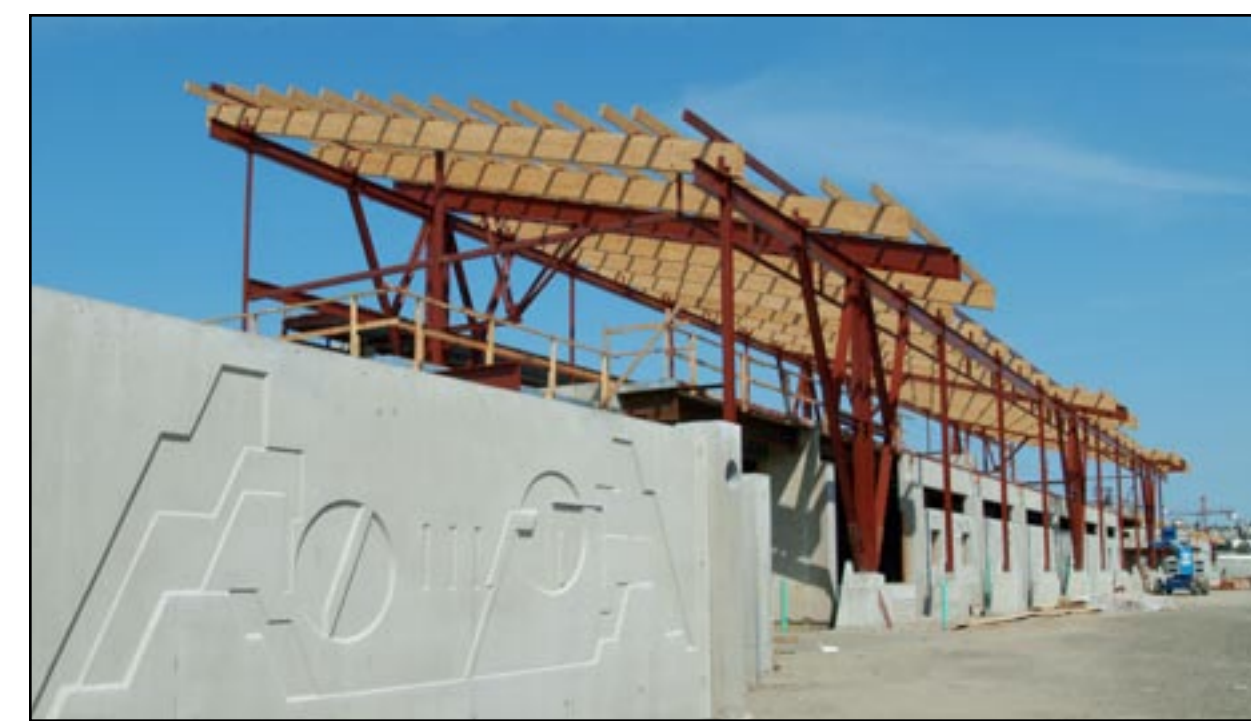
ADMINISTRATION BUILDING UNDER CONSTRUCTION
