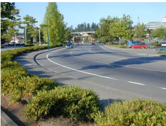
New 3-lane cross-section of EWRR with bike lanes, converted from 4 lanes. Photo: courtesy of City of Surrey.
