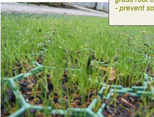
Structural Grass (filled with topsoil and seeded)
