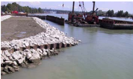
Work on Fish Habitat. Source: Westmar Consultants Inc. and Keystone Environmental.
