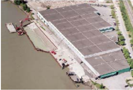
Meadow Avenue Site Nearing Completion. Source: Westmar Consultants Inc. and Keystone Environmental.
