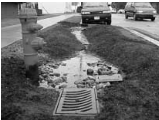
Figure 2 – Infiltration bulge, before planting
